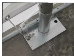
Installation of Back Panel Cover
