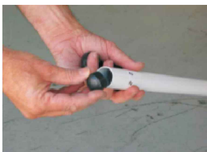
Installing end plugs
