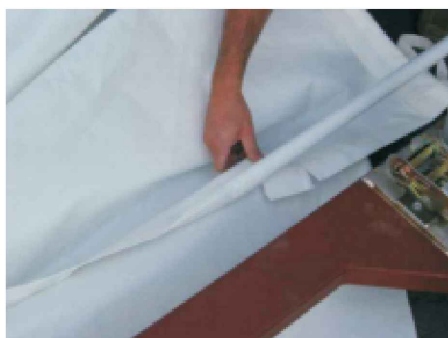
Insert tensioning tubes
