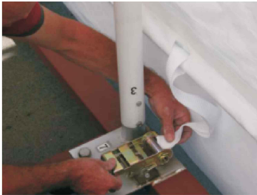
Installing ratchet straps
