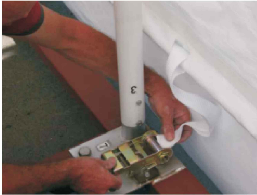
Installing ratchet straps
